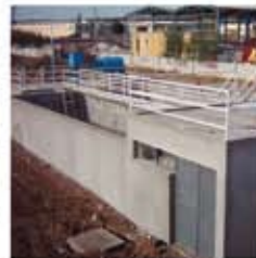
betonarme / reinforced concrete
